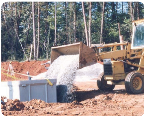
Place gravel in the enclosure and around the side. Lift enclosure to let gravel run underneath.
