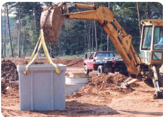
Lift and position enclosure with backhoe.
