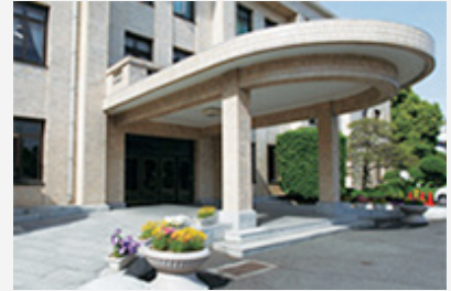
The main building at the Gunma Main Plant provides accessibility with wheelchair ramps
