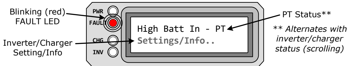
Figure 10-9, PT Controller Fault Message (Example)
