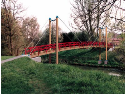
A CINEMA 4D object (the bridge) fits neatly into both a foreground and a background image (scene by Joachim Hoff).
