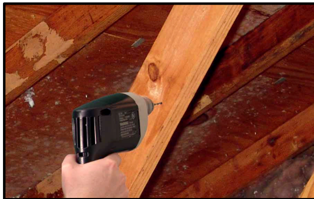
Figure 5 - Drill two holes for mounting bracket
