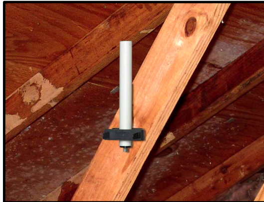
Figure 7 - Secure Signal Antenna to bracket
